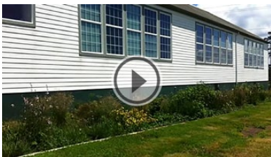
This video does a great job of documenting the installation, function and maturation of this OFG.
